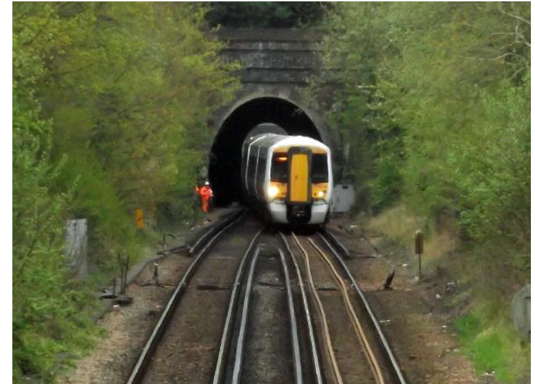
Two tracks become one. Somer Hill tunnel in Tonbridge, one of four single-line tunnels on the Hastings branch
