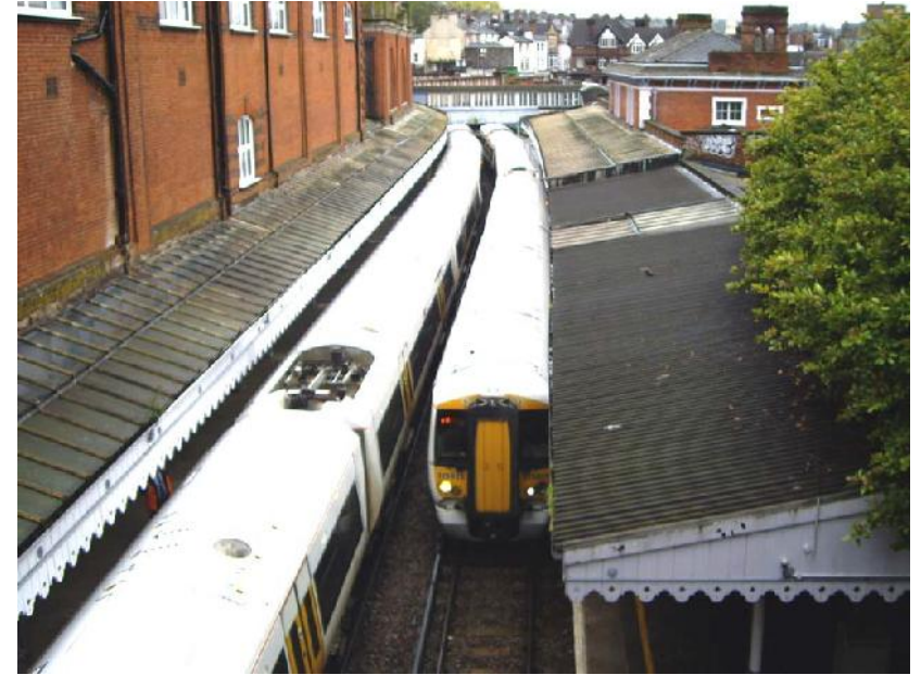
The SER 2-platform Tunbridge Wells station on the Hastings branch remains cramped and operationally difficult
